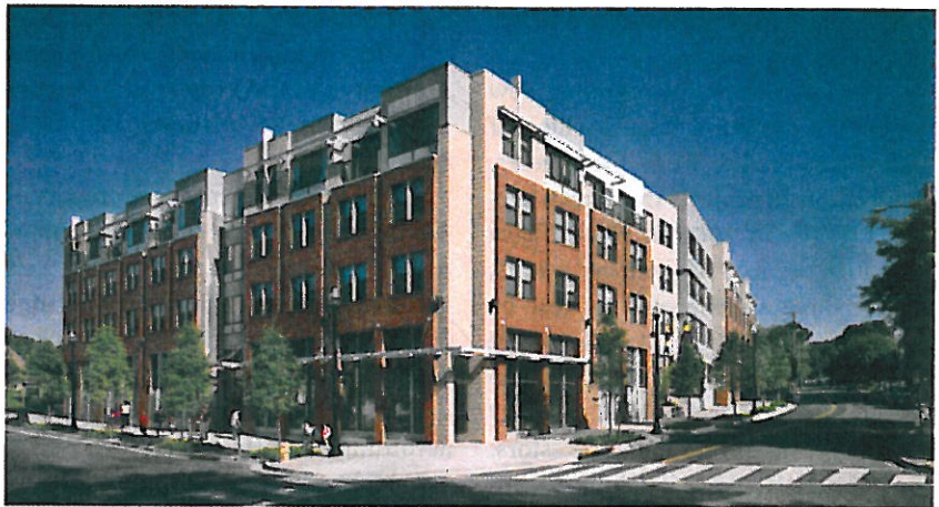
The Shelton earned an honorable mention this year in the metropolitan housing category of the Affordable Housing Tax Credit Coalition's Charles L. Edson Tax Credit Excellence Awards. (Bonstra/Haresign Architects; Photo by Anice Hoachlander)
